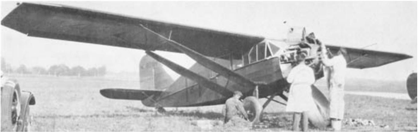
**Bellanca #14. The ring cowling for the J6-9, seen lying on ground, was poorly installed and caused delays during the tour. Note mechanic using bucket for work stand.**
