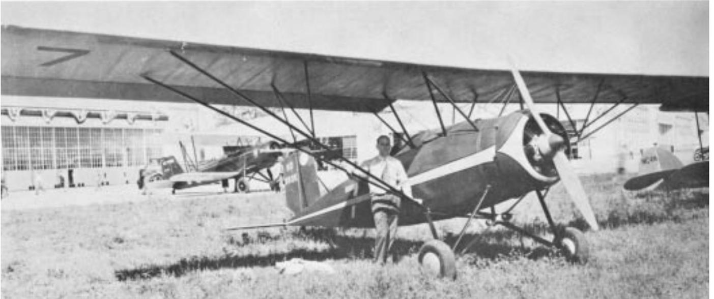
Harvey Mummert and Mercury Chic. The Chic had an unusually high parasol wing, which made it difficult to handle on the ground, and full span ailerons, actuated by push-rods which slanted out through cockpit coaming.
